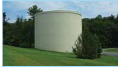
Hospitals & Airports Danville, PA ▶ 1.07 MG TES Tank
