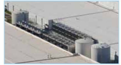
Data Centers Ashburn, VA ▶ (3) 0.50 MG TES Tanks
