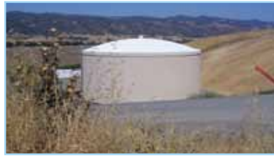
Industrial & Commercial Brooks, CA ▶ 1.37 MG TES Tank
